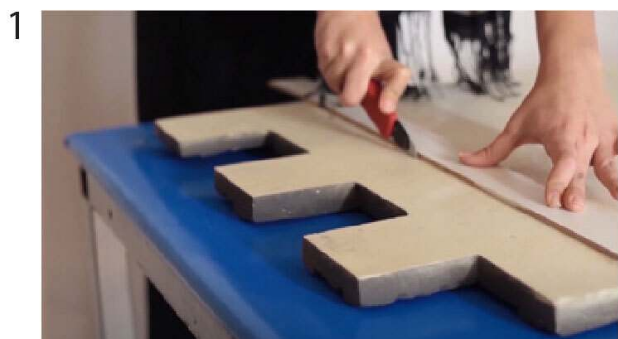
Use a utility knife to cut the panel to fit the wall.
