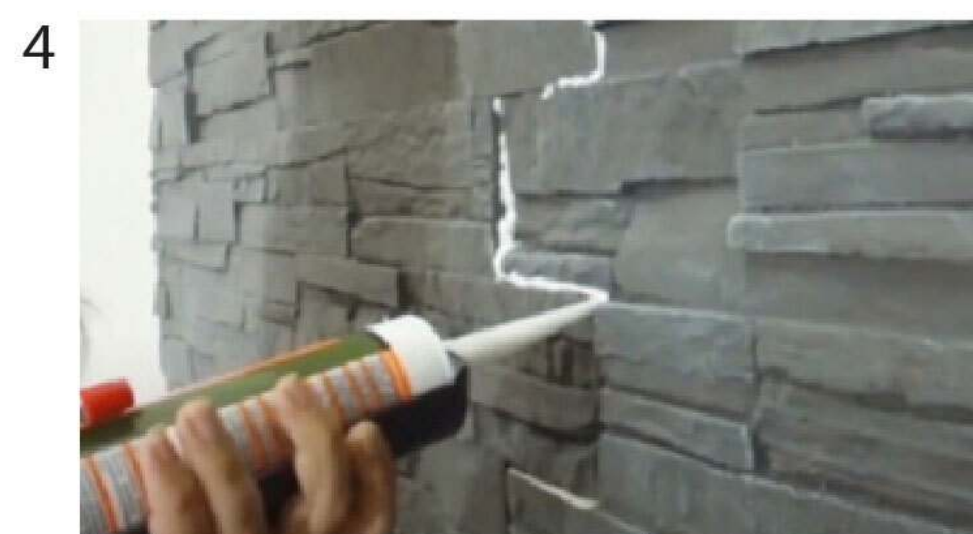
Apply sealant to the joints of the panels.
