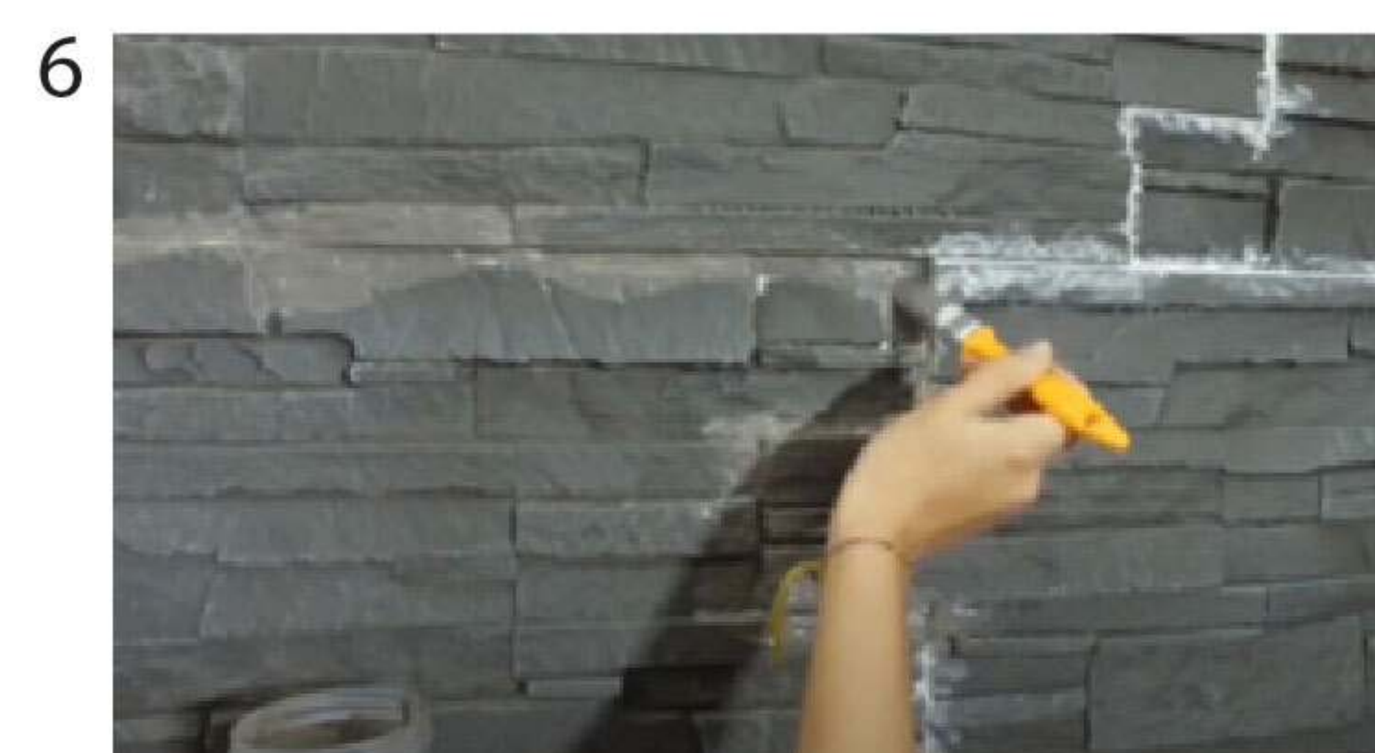
Apply touch-up paint to the dried paste.
